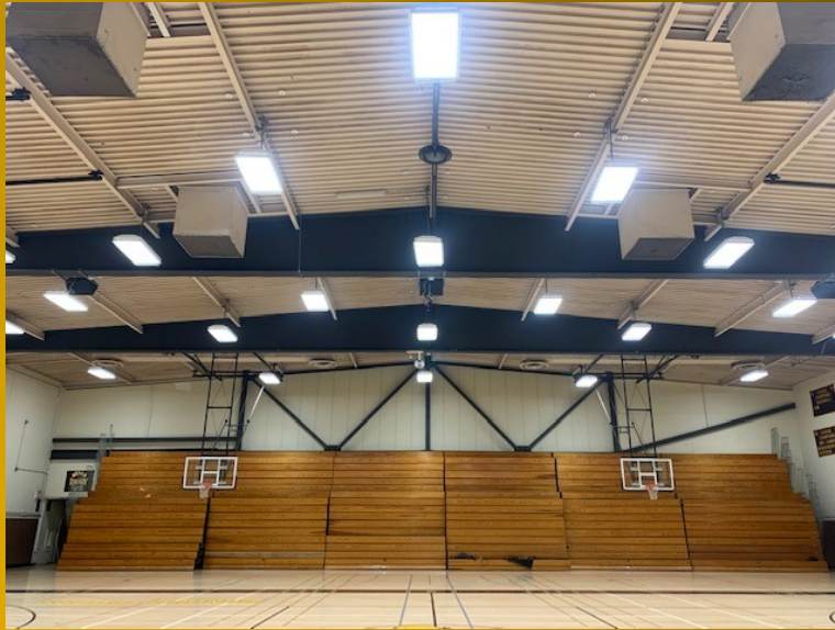
Performance Gym Ceiling
